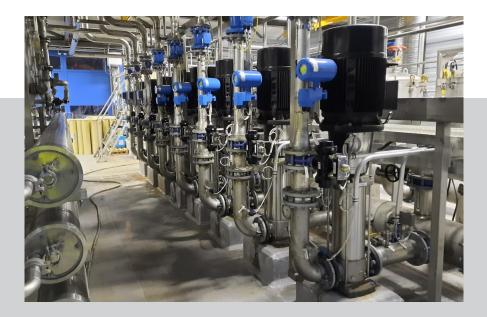
IoT and Electric Signature Analysis (ESA) provide an option to improve both these aspects radically. ESA uses pump motor current measurements to calculate various parameters, such as flow rates and motor usage. This allows for a new way to gain information on the state of pumping processes across operations.
